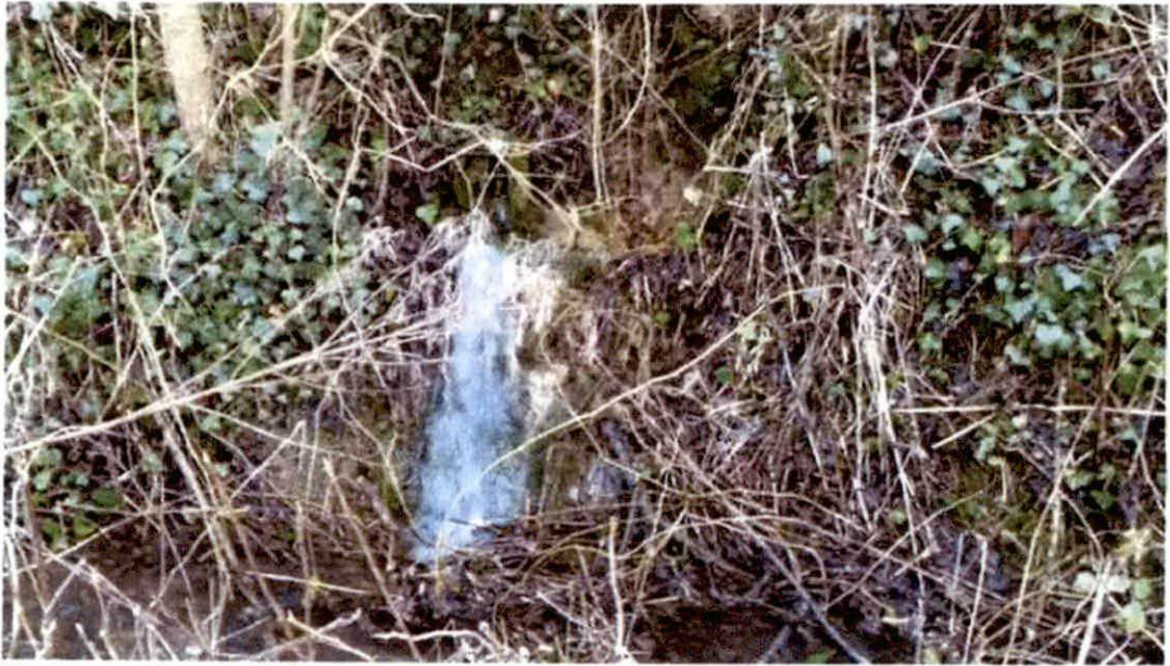
Figure 1: Evidence of flows from land drainage system into ditch on Bell Lane
